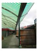
We are satisfied that the lightweight structure remains in good condition and remains structurally stable. Excessive wind loading could cause damage to the canopy and the structural frame in the future although we recorded no evidence of this occurring previously.
