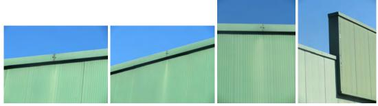
The claddings externally to the elevations and the parapets are clearly aged and the colour is deteriorating, and water penetration has occurred to the soffits as a consequence of leaks to the roof and parapet capping's, as illustrated below. Replacement of the external claddings, whilst not essential, is strongly recommended.
