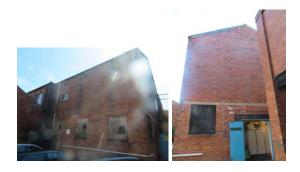
The overall condition of the brickwork is poor, although in general we are happy that the building holds good alignment with little evidence of any undue movement or deflection and we are satisfied therefore that it remains structurally stable.
