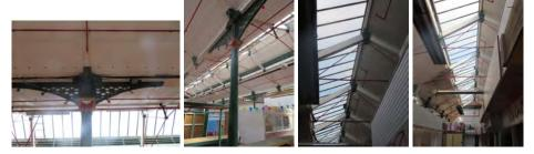
Within the building ventilation and north lights have been incorporated as part of the original design to provide natural light into the unit, as illustrated by reference to the following photographs.
