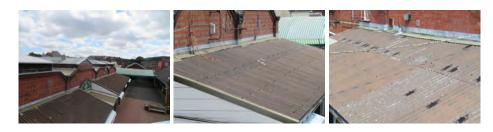
The roofs are structured, it would appear, by precast reinforced concrete portal type sections as illustrated by reference to the following photograph. The rafters and presumably intermediate purlins, which were concealed from view at the time of our inspection, are likely to be of similar formation, generally held good alignment with little evidence of any undue movement or deflection and we are satisfied that they remain structurally stable.
