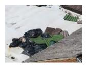
Many of the flashing details at junctions of abutments and intersecting roof pitches are poorly formed and we have highlighted water ingress and repairs which have been undertaken in these areas. Replacement of all flashing details is necessary, in our opinion, and works of this nature should be undertaken in the relatively near term.
