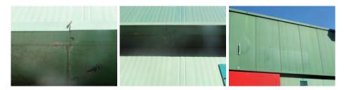
The internal claddings forming sections of these parapets generally appear to be of reasonable condition and given that these are visible immediate replacement is not essential, although as part of the overall renovation and refurbishment of the site amendments to the detailing and replacement of the internal cladding panels may well be considered prudent.
