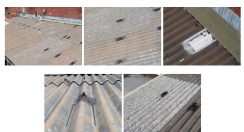
Deterioration to the extremity of the asbestos sheets however was evident below. In our opinion removal of the asbestos cement weathering's are recommended. The works should be undertaken in a controlled manner by licenced contractors and the asbestos material disposed of to a licenced tip. Works of this nature are not of the most urgent form but, in our opinion, it would be good management and appropriate to remove all asbestos components and asbestos cement sheeting from the site.
