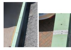
Externally to the elevations there is clear evidence of staining to the cladding panels, as a consequence of water penetration through these joints as illustrated below. Replacement of the capping's is therefore warranted.
