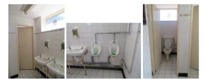
The pipework supplying the facilities is generally corroded and deteriorated due to condensation issues given the absence of any thermal insulation and heating within the toilets as illustrated below.
