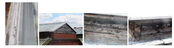
In our opinion complete redecoration of all normally and previously painted surfaces must be contemplated and undertaken within the next 12 months. Failure to apply decoration to timber and ferrous components in particular much increases the risk of rot and corrosion and foreshortens the life expectancy of individual components. Deterioration has occurred due to a lack of regular redecoration and is now necessitating repair and maintenance to many of these such structures.
