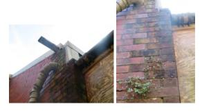
Alterations have been undertaken to the main drainage from the roof and pipework has been run from existing sections to discharge crudely onto hardstandings to the rear of the building, as illustrated below.
