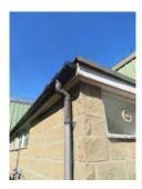
The gutters are aged and a little choked with debris, as illustrated by reference to the following photographs, however in general they remain serviceable at this time. Replacement of the uPVC guttering must be anticipated within the relatively near term.
