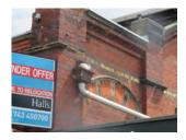
This much increases the rainwater flow onto the flat roof of the hairdressers which is discharged to perimeter guttering, which has generally failed with leaking sections evident, which is likely to have caused deterioration to the fascia and soffit details above as illustrated below. Replacement of the rainwater goods to the hairdresser is recommended and similarly works to the outlet from the front roof and the replacement of the pipework should also be considered.
