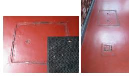
Dampness was recorded within the floors and it is possible that the bitumastic coating was applied originally to limit penetration. It is unlikely that any significant damp proof course was incorporated as part of the original construction of the market, however we cannot confirm our suspicions in this regard.
