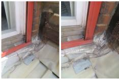
Other crudely formed details are corroding and likely also to result in water penetration due to the limitations in the flexibility of this material, as illustrated below.
