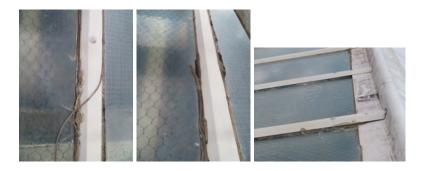
The glazing incorporates many sections of different wired glass, as well as the perspex components. In our opinion replacement of all perspex with new Georgian wired sections is strongly recommended. A number of cracked and broken panes were also identified and these should also be replaced.
