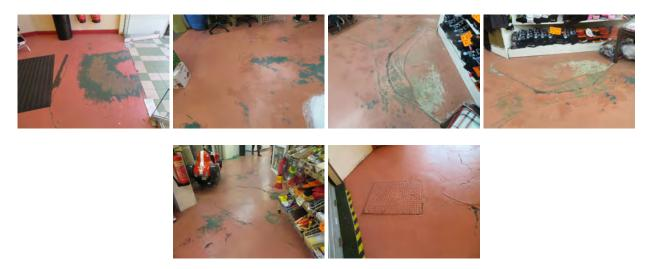
Within the floor cracking and uneven surfaces are identified by warning tapes, as are raised ironworks to inspection chambers forming part of the drainage system, which are also located in the floors as illustrated below. In our opinion whilst the warning tape is of benefit this does not indemnify the owner against claims if somebody were to trip or fall.
