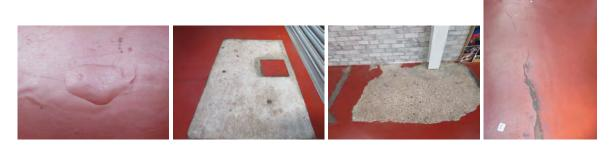
There appears to be a thin bitumastic covering on top of the concrete, as illustrated by reference to the following photographs. Further investigation as to the nature of the floor construction in this regard is required. It is possible that the floor paint which has been applied over the bitumastic coating is beginning to degrade. This treatment is not suitable for a bitumastic sub-base.
