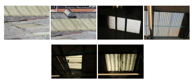
The bolt fixings which secure the sheets to the metal frame are generally aged and corroded and missing caps were recorded, which will hasten deterioration and also facilitate water penetration.
