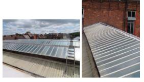
The north lights are timber framed and generally remain in fair condition, however more recently plastisol coated cappings have been introduced to weather timber sections of the roof lights, which may well be rotten beneath the cappings, although these could not be inspected and therefore we cannot confirm our suspicions in this regard.
