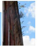
Continued deterioration to the stonework is inevitable and growth of plants, particularly buddleia, is likely to result in the destabilising of the structural integrity of the parapet coping stones and the masonry cornice. The risk of spalling stonework from the cornice is significant and immediate repairs are warranted. Removal of the plant growth is essential and thereafter repairs to spalled stonework and repointing of the joints to the coping stones must be anticipated.
