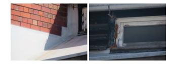
Internally within the property we recorded evidence of water penetration causing staining to ceilings and areas beneath this roof, suggesting that water penetration does occur as illustrated below. In our opinion the detailing is poorly formed, and recovering is strongly recommended.
