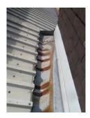
Flashings and crude fixing details at junctions of the vents were also recorded and again these could potentially result in water penetration. Some impact damaged and dented sheets were recorded, as illustrated below but in general the main covered areas of these sections of the roof remain watertight.
