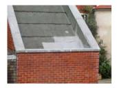
Parapet walls generally held good alignment with little evidence of any undue movement or deflection and on this basis therefore we are satisfied that these remain structurally stable. The lead capping's are in good order however deterioration to the inner felt linings are to be anticipated, as these are aged and were not originally of the highest quality.
