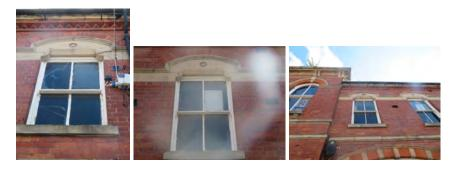
The windows remain in fair condition but are generally aged and single glazed and as such prone to condensation. A lack of decoration is resulting in decoration to the timber framework. Larger windows of this type exist to the rear of the building, as illustrated below.
