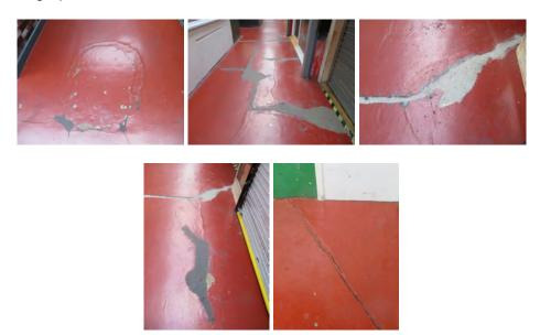
The coating in some instances is also beginning to deteriorate and in other areas it has been removed, as illustrated below.
