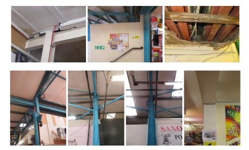
Many of the columns were concealed from view and enclosed within linings and forming sections of the shops and could not be inspected in detail. Where visible they generally remained in fair condition, however we did record some slight evidence of corrosion close to the junction with the ground floor slab, as illustrated by reference to the following photograph.
