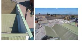
The sheeting remains in fair condition, however we recorded evidence of cut edge corrosion and failure of the Plastisol coating to the edges of many of the sheets, as illustrated by reference to the following photographs.
