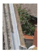
The design of the parapets is however poor and the brick on edge detail is not adequately weathered and is allowing saturation to occur during periods of heavy rainfall. To the external face it is clear that saturation of the brickwork to the flank wall occurs, due to the poor capping detail as illustrated by reference to the following photographs.
