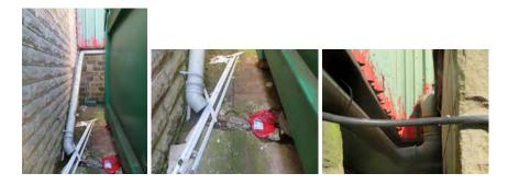
This suggests that either additional drainage has been provided or that the underground drainage system which originally would have collected rainwater from these pipes has failed, or is blocked, and cannot be repaired.
