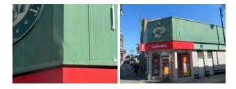
The cladding to the rear area close to the car park or external stores area is badly impact damaged and the decorative coating has failed, as illustrated below. Replacement of this cladding is strongly recommended.
