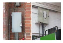
In some areas isolated fuseboards were identified serving individual units, as illustrated by reference to the following photographs. In overall terms the electrical infrastructure is believed to be serviceable but far from being compliant with current standards and significant upgrading and improvement is to be expected.
