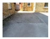
To the rear area, which we believe form parts of the demise, tarmac and concrete surfaces are deteriorating which expose old cobbled sections beneath, as illustrated by reference to the following photographs. Complete reformation and resurfacing of these areas are strongly recommended and should be undertaken in the near term.
