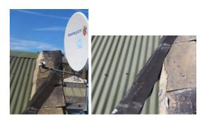
The parapet is misaligned and leans inwardly and the stone copings are clearly facilitating water ingress and some crude repairs have been carried out previously, although in our view these are unlikely to be effective.
