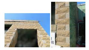
A number of window openings have been blocked up, which is of relatively crude formation, as illustrated by reference to the following photograph. Repairs in this regard are strongly recommended.
