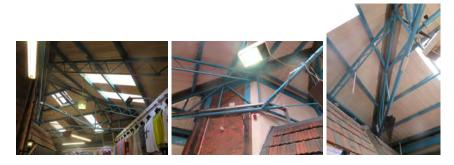
The lattice beams have limited connections and ties but generally held good alignment with little evidence of any undue movement or deflection, as illustrated below.
