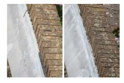
In our opinion the introduction of lead cappings dressed over the brickwork and finished with a welted drip down onto the lead flashings or clear of the building to its extremities is strongly recommended. Works of this nature should be undertaken in relatively near term.
