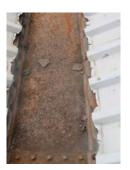
Failure of the mastic joints and the bolted sections can also result in leaks internally.
