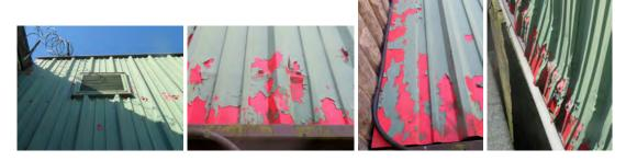
Replacement of the cladding systems may well be required in due course, although despite their age and minor damage it is our view that these remain serviceable at this time.
