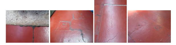
At present the floor remains serviceable, however the coating is likely to become slippery when it is wet, and the overall condition of the floor is deteriorated. Excavation of the bitumastic base may well be required and the use perhaps of a non-slip resin finish would be of significant benefit.
