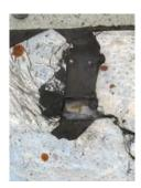
Older lead flashings weather junctions with the vents to the main north lights and these are split, crystalline and in very poor condition as illustrated below. Replacement of these lead details is also necessary and should be undertaken in the near term.
