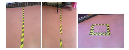
The overall conditions of the floor slabs are poor, in our opinion, and extensive remedial works and the introduction of new non-slip coverings are strongly recommended to return these to a sound, level, safe condition. Complete restructuring of floor slabs throughout the indoor market may well be required.
