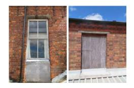
The base of the door leading into the xxxx building to the left hand side is extensively rotten due to leaking gutters and down pipes and neglect previously and replacement is therefore warranted, as illustrated below.
