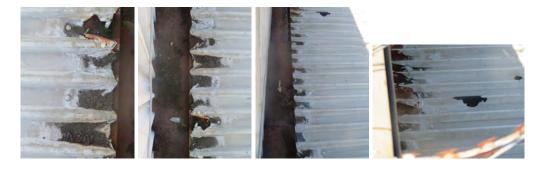
At present the Plastisol coated detailing remains serviceable, however its overall condition is deteriorated and cut edge corrosion, if allowed to persist and develop further which will be the case, will result in corrosion and perforations within the sheets which will clearly allow water penetration to occur.
