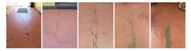
The floor appears to be covered with a bitumastic based material, possibly to prevent rising and penetrating dampness.
