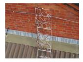
Holes have been drilled in the flashings to allow cables and wiring to serve the Christmas decorations to be introduced. Clearly this is not ideal and increases the risk of water penetration in this location.
