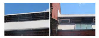
The quality of workmanship is generally poor in our view with detailing at abutments of brickwork and timber clad sections poorly applied and liquid coating sections added, as illustrated below.
