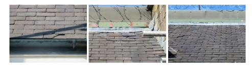
The lead flashing details at the abutments of the stonework and the clad rear parapet are poorly formed and could result in water penetration, as illustrated by reference to the following photographs.
