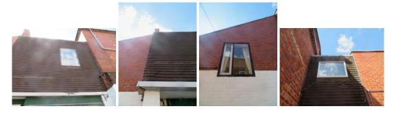
The quality of the build was not of the highest order and subsequent maintenance is poor, with much damage evident to vertically hung tile sections, as illustrated by reference to the following photograph. A systematic and focused renovation and refurbishment of these external areas will improve their overall condition.
