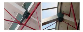
Our inclination is that the main roof structure remains in good order and certainly without evidence to the contrary we cannot recommend significant replacement. It is likely also that the structure and design may well be listed. Further intrusive investigation, testing of the component strength of the metal framework and ties is recommended to ensure that these remain in serviceable order, as we believe to be the case.
