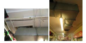
We cannot confirm if the system is operational, although we anticipate as a minimum that much maintenance will be required. Servicing of the mechanical ventilation system should be carried out by a specialist contractor and assessment of its necessity and adequacy undertaken. It is likely, in our opinion, that complete replacement of this is required.
