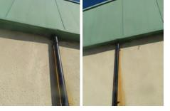
The downpipes discharge directly into open gullies located within the pavement area, as illustrated by reference to the following photographs. This is not ideal in our view and the downpipes could potentially be damaged and also these could represent trip hazards for pedestrians.
