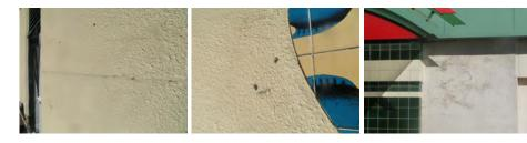
The latter photograph illustrates saturation and dampness due to leaks, which is causing a deterioration to the render surface. Repairs and perhaps complete re-rendering of the flank elevation must be anticipated within the foreseeable future. Clearly continued saturation due to defects in the roof will exacerbate matters in this regard.
