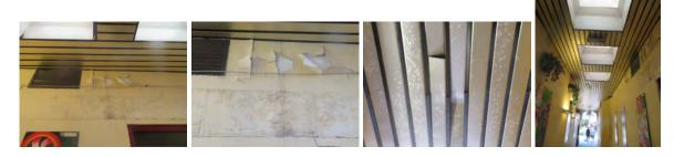
It is likely therefore that the roof is approaching the end of its useful life and recovering is required. Given the water penetration the likelihood of rot to the deck and structure is high and replacement of much of the structure should therefore be anticipated.
