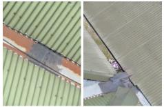
Internally sections of the box gutters were evident and also exhibit corrosion suggesting that the box gutters are approaching the end of their useful life, as illustrated below.
