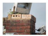
To the rear corner it appears a section of the parapet has partially been taken down and is of a single half brick thick formation, as illustrated below. The felt weathering's have been applied, which are generally of poor formation, and improvements in this regard are strongly recommended.
