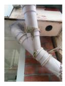
Similar crude pipework also runs from other box gutters close to the hairdressers, as illustrated below. Rainwater in this regard discharges in some instances directly onto the hardstanding and is not adequately collected and disposed of.
