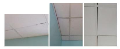
Within the plant rooms plasterboard ceilings have been formed and attached presumably to the underside of a timber frame. The ceilings are not skimmed to a finish, however there is no concern in this regard.
