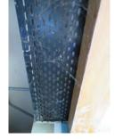
The use of these lintels is in keeping with building practice at the time the property was constructed and in general they provide adequate support and we are satisfied that the window openings remain in good order. The absence of any significant movement to the window arches reaffirms our assessment of the overall structural stability of the building.
