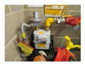
Gas supplies are generally restricted to within the plant room and appear to be in good order with no evident gas smells recorded at the time of our survey. Testing of all gas fired appliances and the provision of a suitable Gas Safe Certificate is strongly recommended and works of this nature should be undertaken in the near term.
