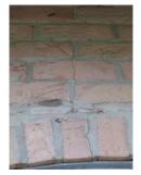
In our opinion this is indicative of thermal expansion. Expansion joints have been constructed within various sections of the property and generally at junctions of return wall, as illustrated below. The mastic seals to the expansion joints remain generally in fair condition at this time, but in due course replacement must be anticipated.
