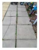
In our view the pavings are in poor condition and represent a potential trip hazard. Replacement of the uneven paving, particular to the main entrance areas is essential and should be undertaken in the near term.
