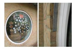
The windows in all other openings are spanned by means of Catnic lintels which provide support to flat brick arches, as illustrated by reference to the following photograph.
