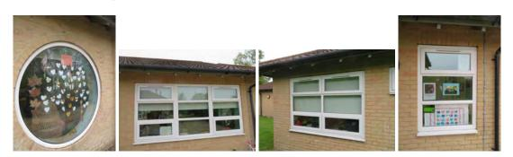
In general the windows remain in fair condition, considering their age and nature. The mastic seals at the junctions of the window frames and brickwork are beginning to deteriorate and could potentially facilitate water ingress, as illustrated below. Replacement of mastic seals should therefore be contemplated as part of general maintenance works in respect of the building.
