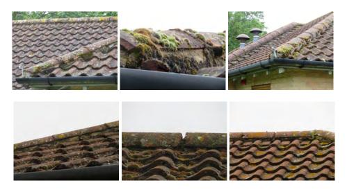
It is apparent that one hip has required works and the tiles have been replaced in this instance, as illustrated below, suggesting that failure of the ridge and hip tiles could well occur during extremely inclement weather. Removal of all ridge and hip tiles, rebedding and repointing is therefore strongly recommended as part of a maintenance programe in respect of the roof.
