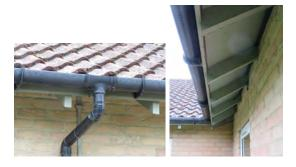
The guttering appears to be the original installation and there is evidence of numerous leaks to joints, as illustrated particularly by reference to the following photographs.
