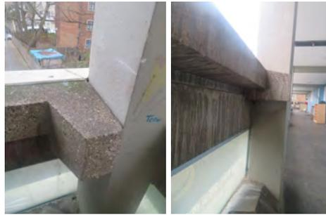
The balustrading to the second floor walkway incorporates a top rail and a bottom rail, with a glazed section set within, as illustrated by reference to the following photograph.
