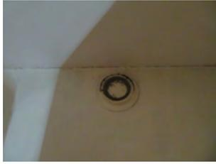
We recorded a mechanical extract fan within the kitchen which is acceptable although it should be upgraded in our opinion. The introduction of modern mechanical extract fans is considered essential, in our view, and ideally these should incorporate a humidistat so that moisture laden air is expelled from the property upon generation. This will assist the reduction of condensation within the flat.
