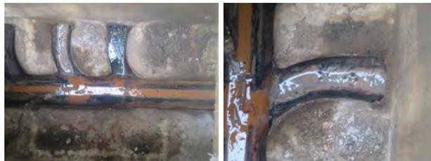
The photographs illustrate a build up of limescale within the pipework and descaling and cleaning of the underground drainage installation is strongly recommended and should be undertaken on a regular basis.
