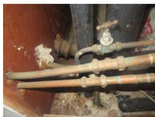
The majority of pipework was concealed from view and could not be inspected in detail; however, we recorded no evidence of leaks or particular defects. Replacement of the supply pipework may well be anticipated in conjunction with the renewal of the sanitary facilities.
