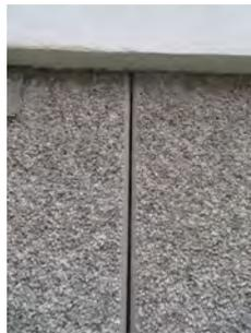
In isolated areas we recorded minor damage to panels, possibly following the insertion of fixings, as illustrated below.
