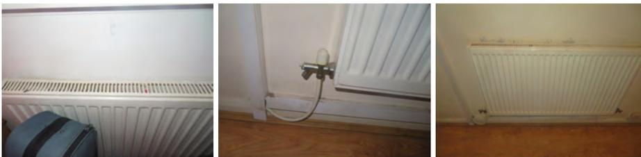
We recorded no particular evidence of defects or leaks to the central heating system, which we anticipate operates adequately. Servicing and overhauling of the system are, however, essential and, in our view, the heat output from a number of the radiators is potentially lower than considered desirable given potential heat loss from the property.
