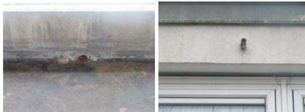
The design of the outlets and the details is somewhat poor and water ingress could occur in these vicinities.
