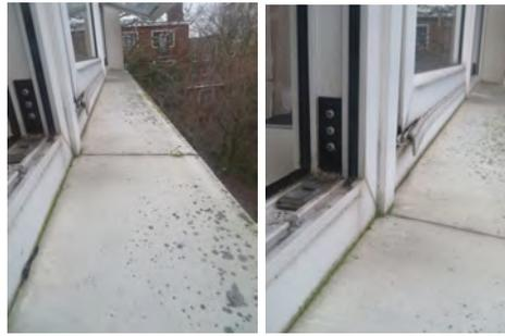
There is evidence of water penetration and deterioration to these capping's, which could undermine and affect the overall condition of the insulation in due course and also cause failure of the render. The trim details and capping's, where these have been introduced in various locations, do not adequately discharge rainwater clear of the render beneath, resulting in saturation in various sections, as illustrated previously and also by reference to the following photograph.
