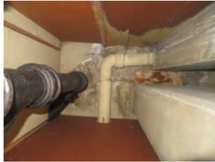
Rainwater from the balconies is discharged via small overflow pipes which, if surcharged, would discharge onto the pavement below. The overflow pipes are illustrated generally by reference to the following photographs and are serviced by internal openings within the asphalt and balcony weatherings.
