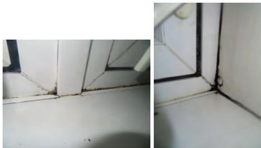
The windows are deteriorated and many of the frames are dirty with corroded fixings and opening mechanisms evidence, as shown below.
