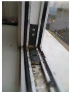
Internally within the flat, many of the restrictor stays, catches and security devices to the windows are also broken, as illustrated below. Similar deterioration is evident in other areas.
