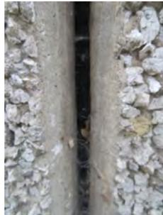
The concrete cladding panels are of pre-cast formation and it is normal for these to be suspended by fixings from the concrete frame. During the course of our survey we were unable to gain sight of any fixings; however, the apparent suspension of panels was evident at low level, as illustrated by reference to the following photograph.
