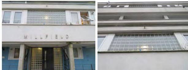
The glass blocks generally remain in fair condition commensurate with their age and nature. The insulation provided by the glass blocks is limited; however, there is no necessity for significant insulation levels to be provided to the common areas, which are generally unheated. The glass blocks remain in fair condition and some repointing may be required over time but, beyond this, significant remedial works are considered unlikely.
