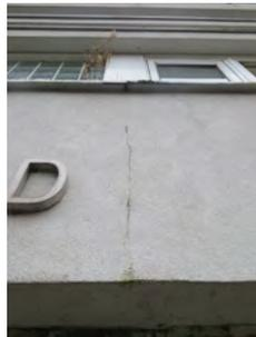
Leaks from boiler flues and overflows have also caused staining to the pre-finished render, as illustrated by reference to the following photographs. Such deterioration may hasten the need to carry out repairs or replacement of the rendering over time.
