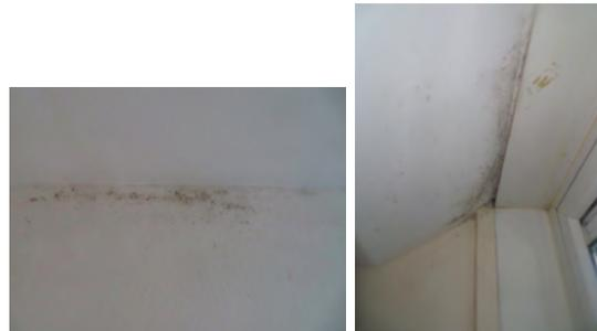
The thermal insulation, where applied to the upper parts and the top two floors, appears to be of more benefit; however, given the fact that the front elevation does not run directly above the floor beneath, the floor at third floor level is effectively not insulated. Lining boards have been incorporated, however, where these have been removed by others and the concrete slab was clearly evident, as illustrated by reference to the following photograph.
