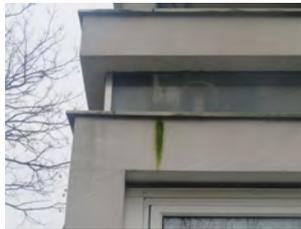
Some weathering and deterioration to the render has occurred and minor sections have been impact-damaged, as shown below.
