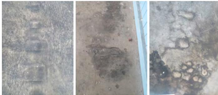
Expansion within the building has also caused rippling or crazing within the asphalt surface which, over time, is likely to result in splits developing and consequential water ingress into the flats beneath.
