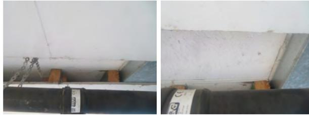
Cracking was evident to the board joints in many areas, as these are not effectively taped but simply close-butted, as illustrated below.
