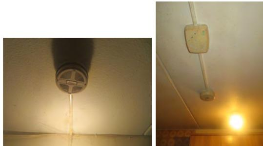
The property has a smoke detection system which appears to incorporate a combined carbon monoxide detector, although we cannot confirm our suspicions in this regard. Our recommendation is to upgrade the smoke detection system within the property, so it is fully compliant with current regulations, and incorporate a heat detector within the kitchen.
