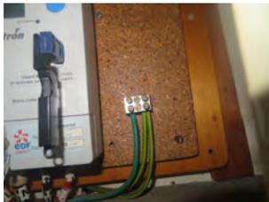
The casing to the mains electrical cables is missing and potentially live wires are exposed, as illustrated by reference to the following photograph. Testing of the system by a NICEIC registered contractor is essential and, in our view, this is likely to identify defects and shortcomings which have been permitted to accrue.
