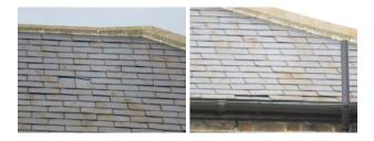
Replacement of broken and slipped slates should therefore be carried out but significant remedial works are not anticipated in the near term.
