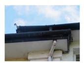
Rainwater from the front canopy roof discharges via an outlet to a hopper which is of basic quality and installation but remains serviceable, as illustrated below. Some improvements are to be anticipated but at present the rainwater goods appear to function adequately.
