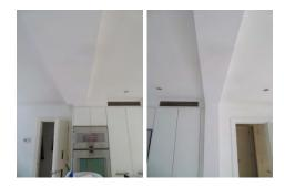
It is likely, in our opinion, that the downstand beams have improved the overall structural integrity of the building and we recorded no evidence which would indicate failure or defects in the works utilised in the implementation of these works. Copies of Building Regulations Approval for the structural alterations would however provide comfort that these have been carried out appropriate, as we anticipate to be the case.
