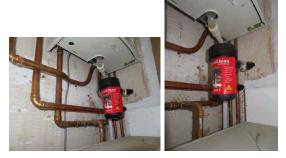
Copper pipework from the boiler runs to distribute hot water to the various radiators located throughout the property which are generally of good modern origin and illustrated by reference to the following photographs. A number of radiators are small in size and not located beneath windows which can reduce their efficiency and effectiveness.
