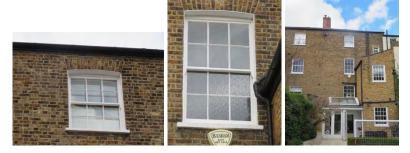
The windows remain in fair condition considering their age and nature; however, there is some evidence of deterioration to window cills which perhaps suggests poor decoration in recent times as well as also basic making good of rotten timber cills, as shown by reference to the following photograph. Overhauling, maintenance and decoration of the single glazed double hung sash windows will improve their overall condition.
