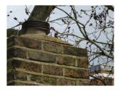
The flashings which weather the junctions of the various chimney stacks and roofs are adequate but not of the highest quality, particularly to the front of the main stack as illustrated previously. Whilst it is not essential reformation of the lead flashings may well be required in conjunction with repairs and repointing and works of this nature should be undertaken in conjunction with future external repairs and redecorations to the property.
