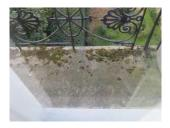
In our opinion, a liquid applied waterproof coating should be introduced to the balcony and the terrace roof to upgrade its integrity to a level whereby it is suitable to prevent water ingress. We recorded no particular evidence of penetration through the underside of the balcony which is supported by means of corbelled brackets, as shown by reference to the following photograph.
