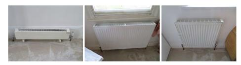
The energy efficiency of the radiators is assisted by modern thermostatic control valves which remain generally in good condition, as shown below. We have not carried out any heat loss calculations and cannot therefore confirm that the heat output from the central heating system is appropriate, as we believe to be the case. Some improvements to the level of output from the central heating system may well be required; however, at the time of our survey the house was very warm.
