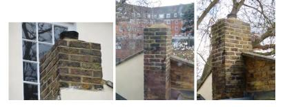
It is clear by reference to the following photograph that the flaunching is cracked as shown below.
