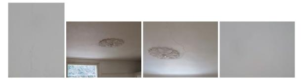
Cracking was also evident at junctions of lath and plaster ceilings and walls, particularly to the rear staircase area as a consquence of movement of the building historically, as illustrated by reference to the following photograph.
