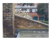
The parapet is weathered by means of concrete coping stones which slope downwards. As often happens with details of this nature rainwater run off is not adequately discharged where the sloping section meets the flat section of the parapet and also due to poor pointing of the joints saturation is occurring of the brickwork beneath, as illustrated by reference to the following photographs.
