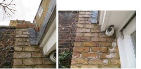
The lead flashings at the junction of the new party wall are generally well formed and remain in good condition. The flashing details to the other parapets are also serviceable and watertight, in our view, and we recorded no evidence of deterioration internally as a consequence of this detailing. It may be prudent, however, in due course to replace the flashings in conjunction with recovering of the various flat roofs which abut the parapet walls.
